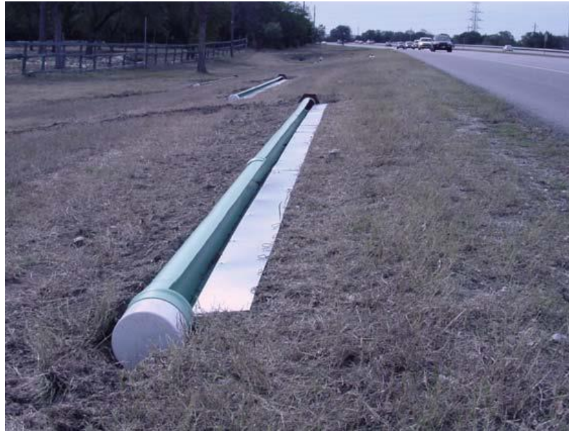
Figure 2-21 Collection Pipe Assembly for First Flush Sampler (Kearfott et al. 2005)
